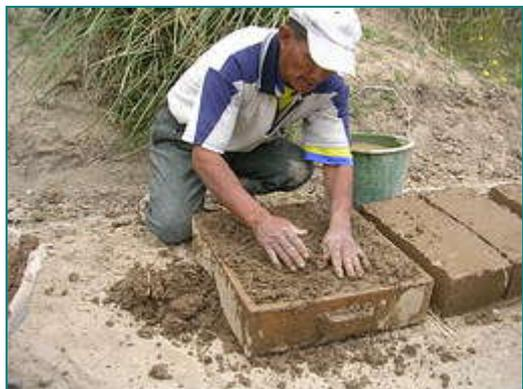
*ADOBES: for the Chugchilán Recycling Centre. Mining clay along the road to hand mix with straw and water.*
